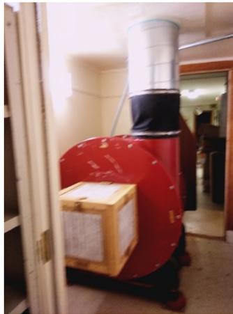
*Figure 27 Air Filter on Intake*
